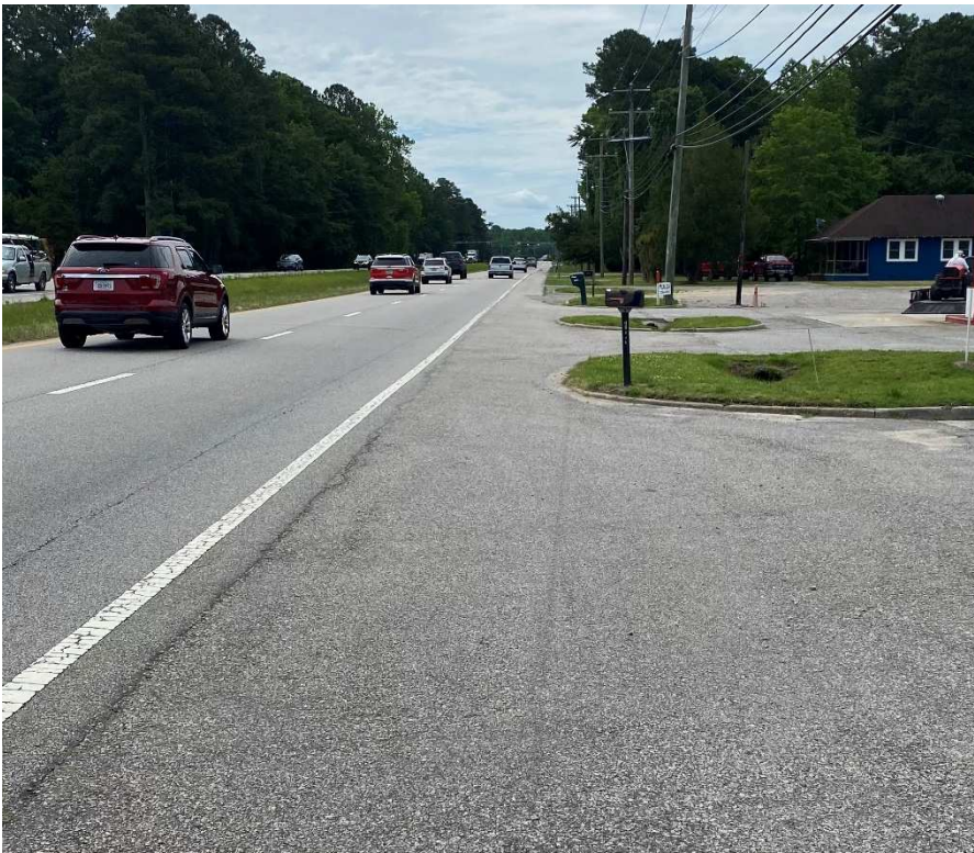
The entrance to the site along Rt. 17.
