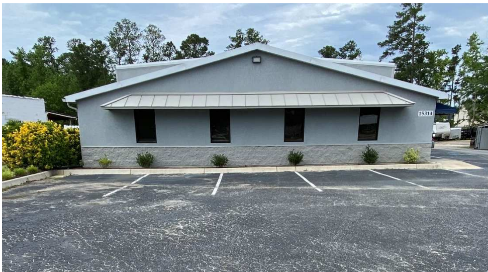
Existing building on parcel 34B-01-012.
