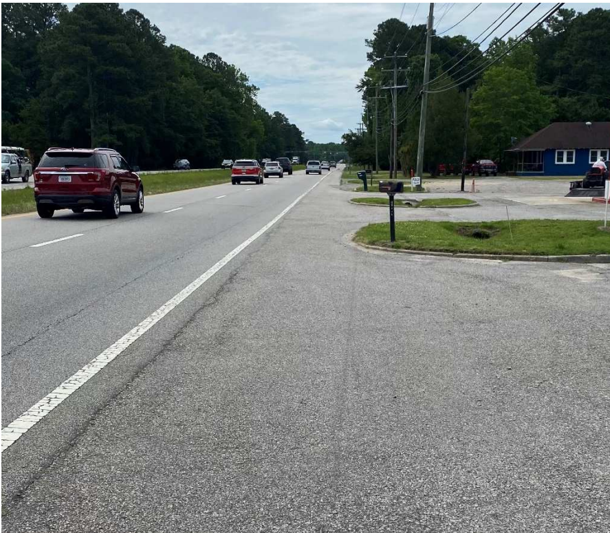
The entrance to the site along Rt. 17.
