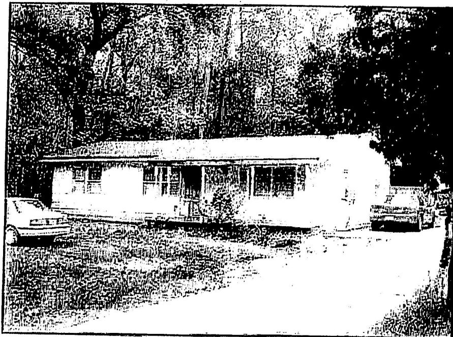
Figure 28. Northeast Oblique of House (Structure 6) at 15366 Carrollton Boulevard.
