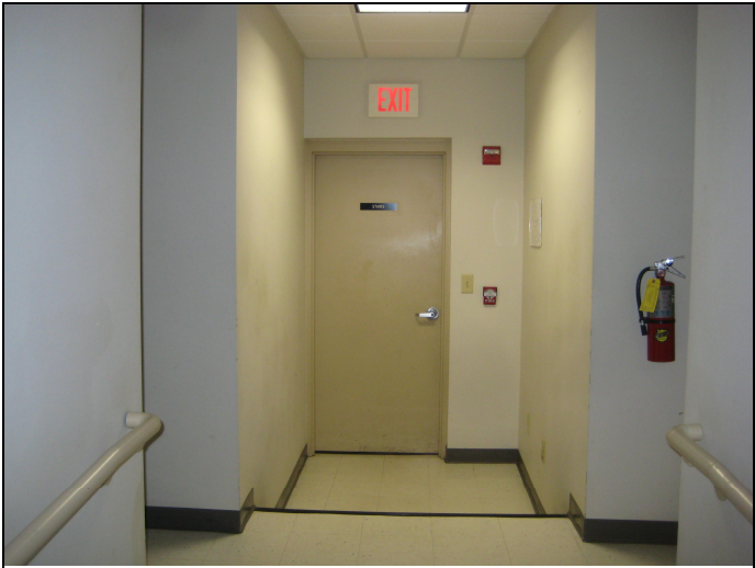
14. Rear exit stair
