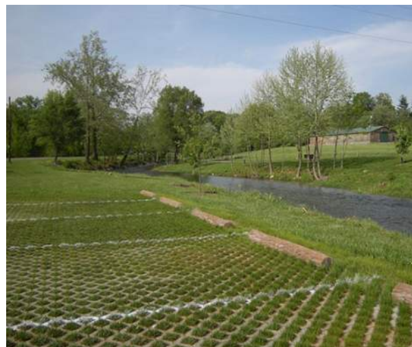
Grass Paver Parking Lot
