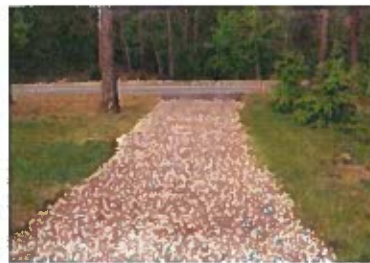
Crushed Shell Parking Lot
