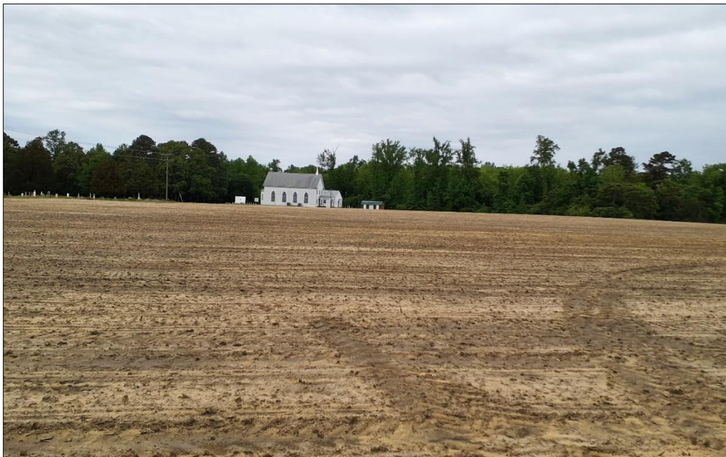
Figure 6-54: View north toward historic church, Resource #046-5154.
