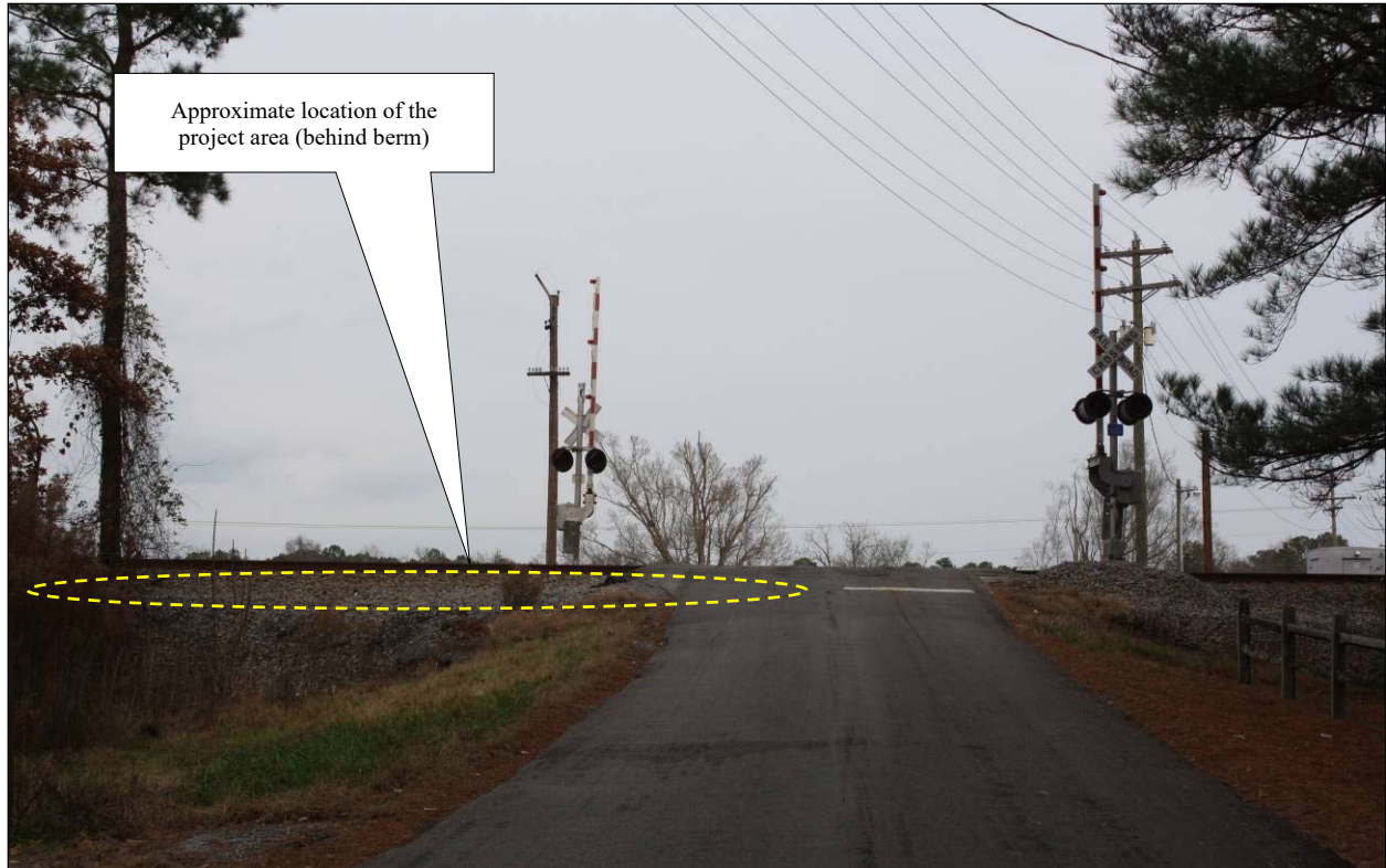
Figure 6-30: View 6- Norfolk Southern Railroad corridor at Antioch Road (project area not visible – screened by raised berm).
