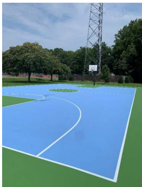
The basketball court at Nike Park was resurfaced in 2023.
