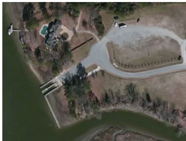
Jones Creek Boat Ramp aerial photo
