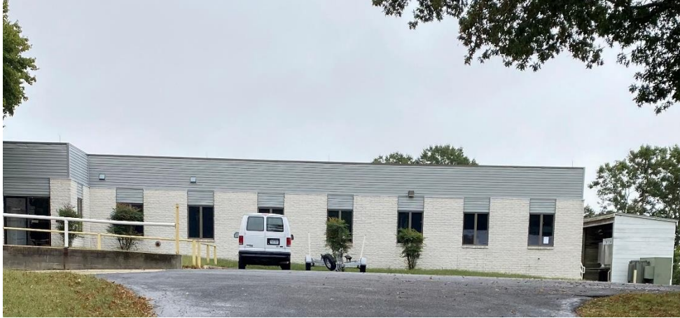
Southern portion of the existing building
