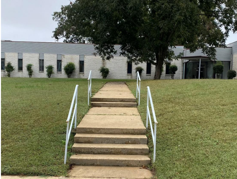
Northern portion of the existing building
