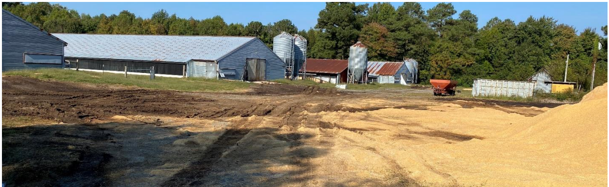
Existing structures on 72-01-022 to be removed if approved
