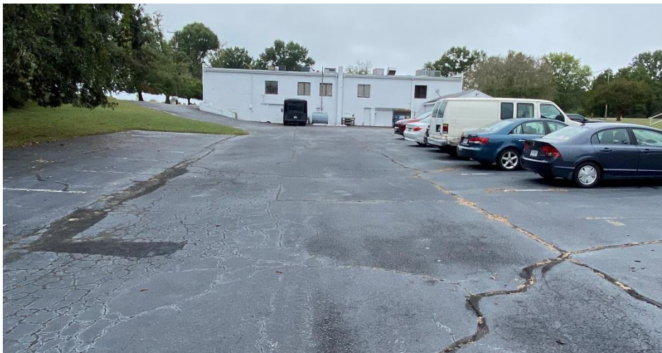
A portion of the existing parking
