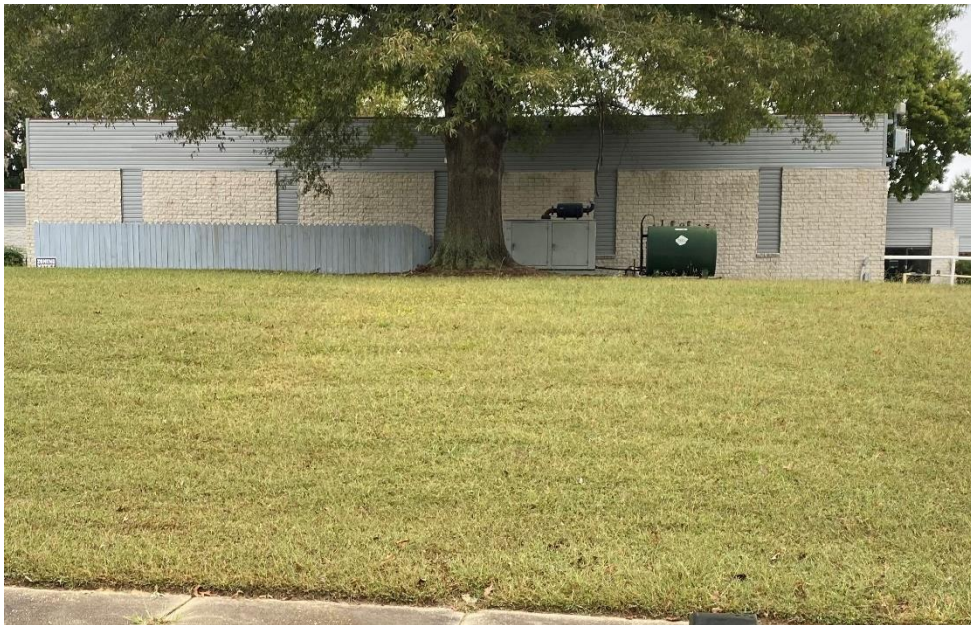
Center portion of the existing building
