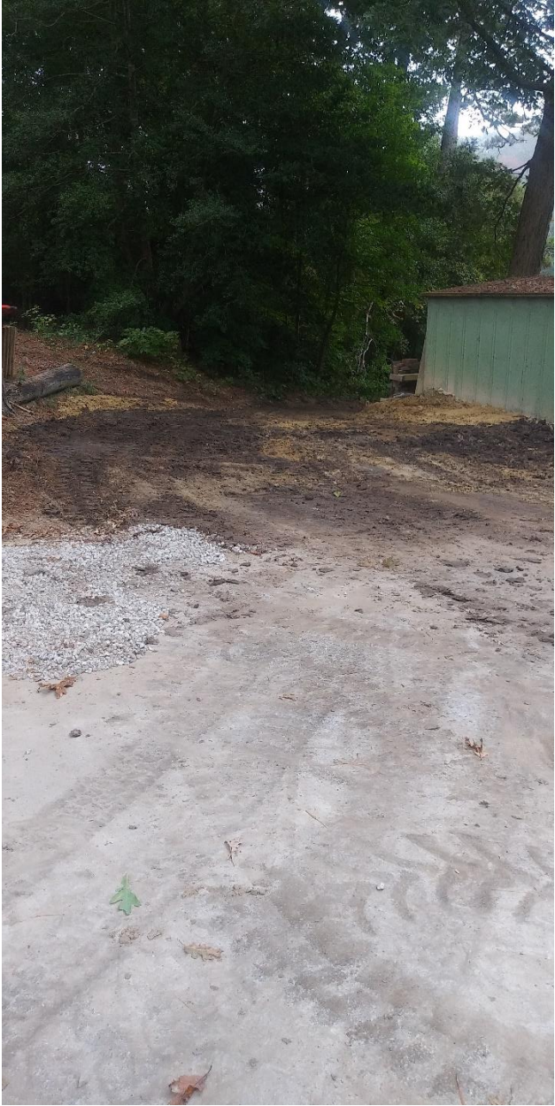
Along side wall
