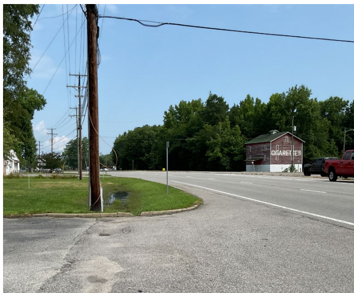
Figure 16. Utility Poles Obstructing Sight Lines from Driveway Looking North of Intersection
