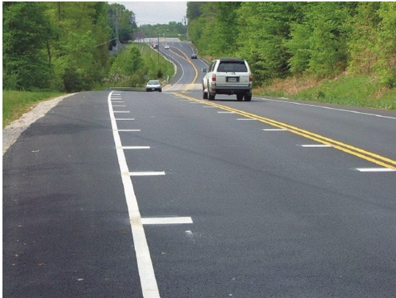
Figure 21. Optical Speed Bar Markings on Roadway (Source: Virginia Center for Transportation Innovation and Research)
